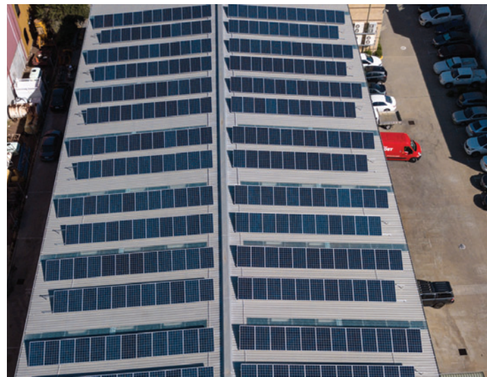
Rooftop solar panels at our pump distribution center in Wangara, Australia.
