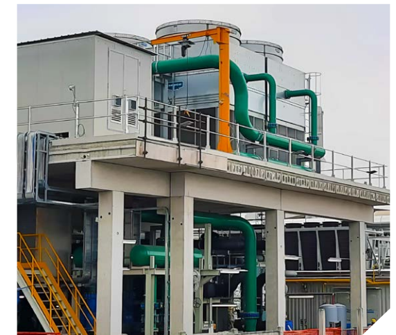
Construction site for Combined Heating and Cooling Power System in Barge Italy
